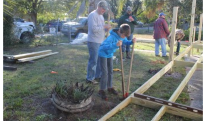
Ramp Building – Lee Taylor, Conner Taylor, B.J. Flores and others.
